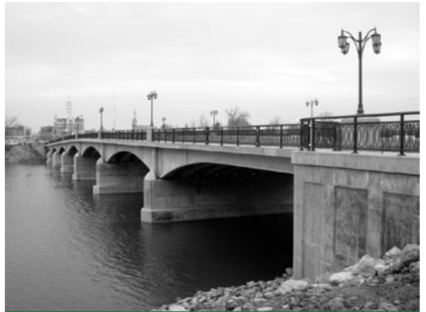
State Route 108 Perry Street bridge in Napoleon.
