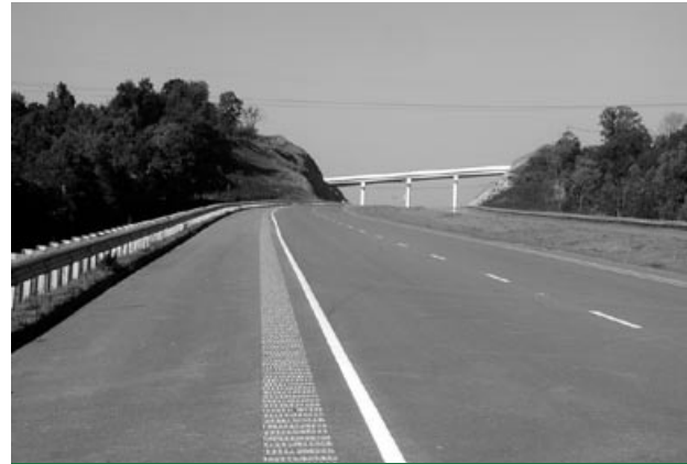
The new U.S. Route 33 Lancaster Bypass.
