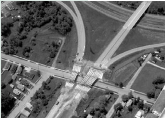
Aerial view of work in progress on the State Route 711 project.
