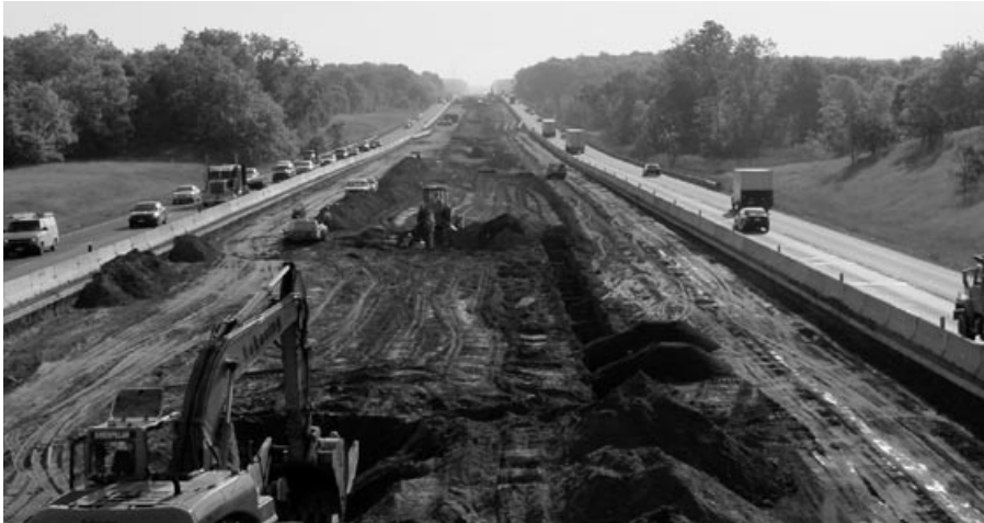
Interstate 71 widening in Medina County.
