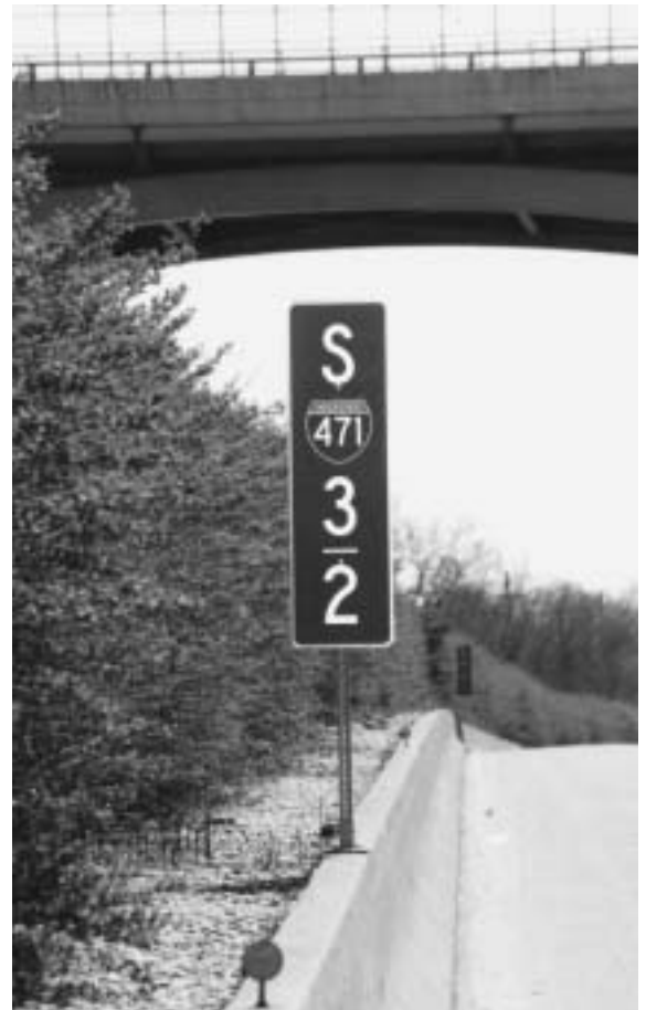
Motorists can use Freeway Reference Markers to identify locations along the road. The signs have been used successfully in Cincinnati since 1995.
