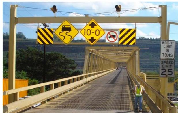
Figure 23 – Excessive Restriction Signing can be distracting
