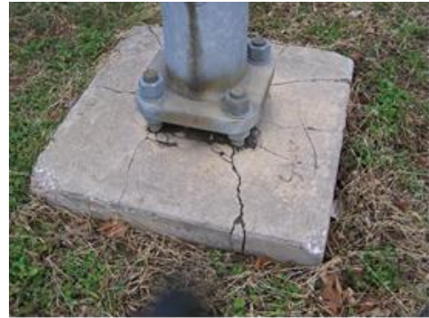
Figure 4.2 Cracked foundation
