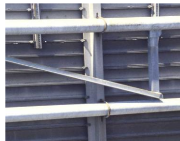
Figure 4.8 Sign attachment assemblies
