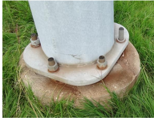
Figure 6.9 Missing anchor nut
