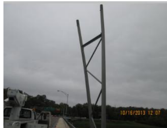
Figure 5.29 Damaged BMS
