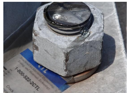
Figure 6.3 Checking for tightness (District 2)
