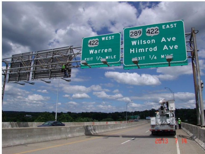
Figure 2.6 Bridge mounted sign (support mounted on barriers)
