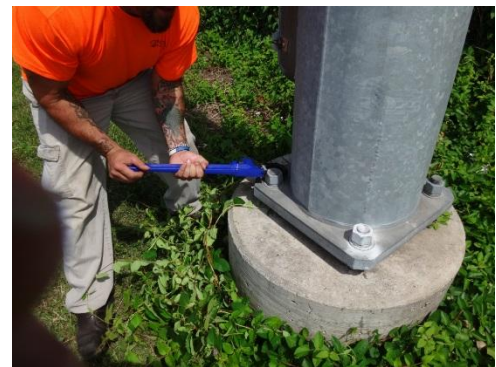
Figure 6.2 Checking looseness of anchor bolt - 24" wrench (District 2)
