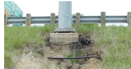
Figure 4.3 Soil erosion
