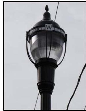
EXISTING WATERVILLE LIGHTING
