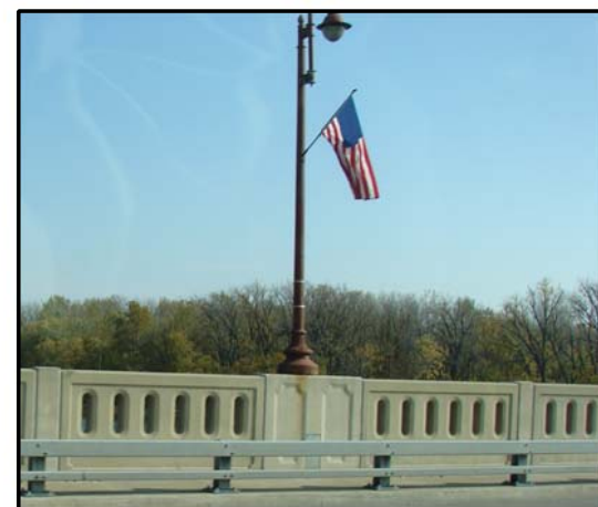
MAUMEE-PERRYSBURG BRIDGE BARRIER/RAILING/LIGHTING
