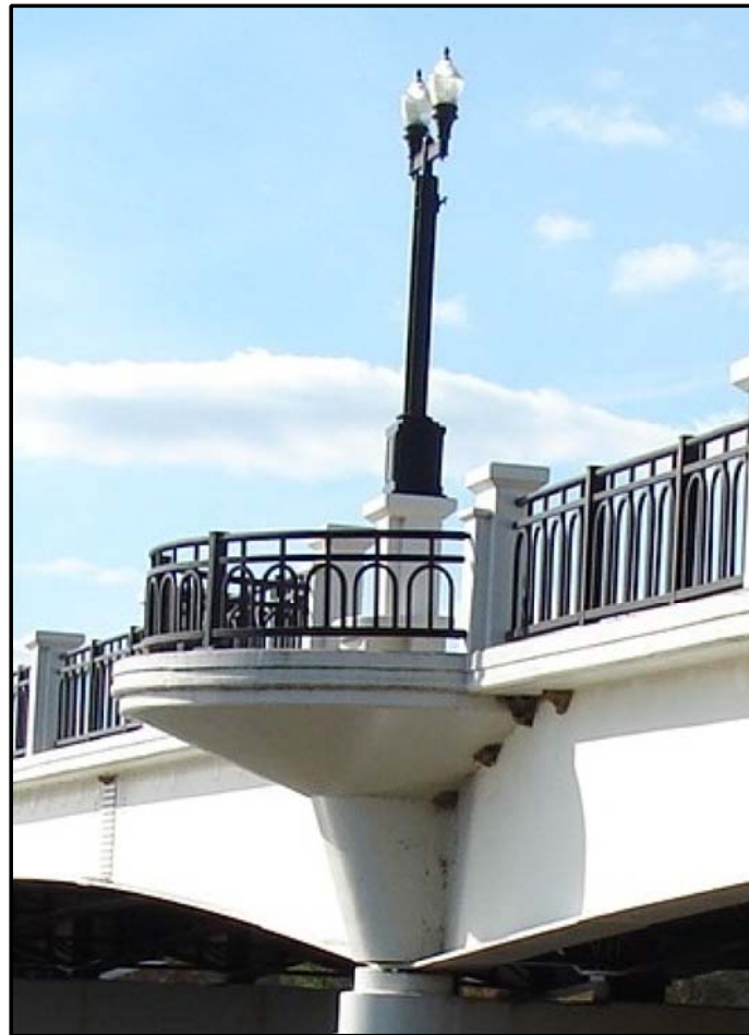
HOME ROAD BRIDGE OBSERVATION PLATFORM
