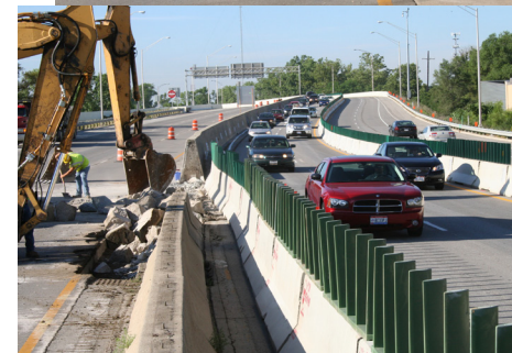
SR 315, pictured above, used crossovers to maintain traffic and access.
