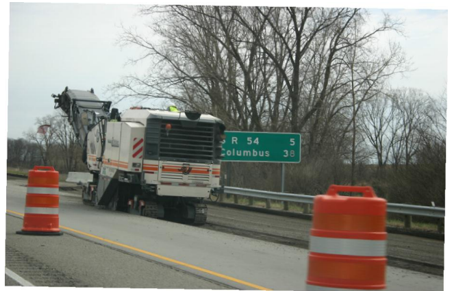
Crews working on the I-70 lane addition in Clark County
