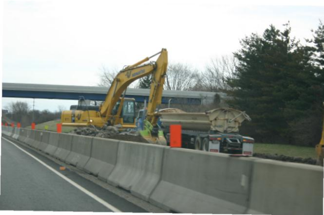
Crews working on I-70 eastbound lane addition
