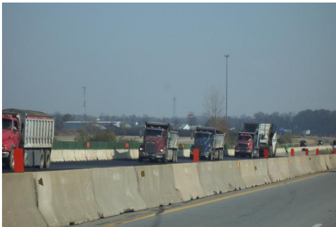
I-70 lane addition in Clark County
