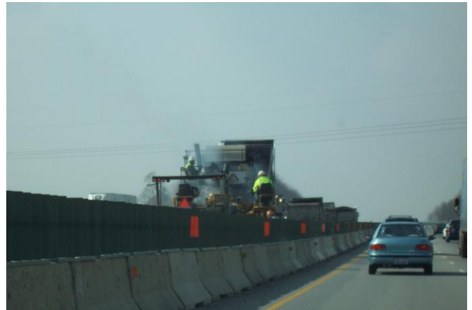
Crews working on the I-70 lane addition in Clark County
