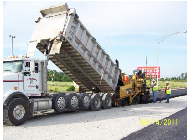
Asphalt placement on the I-70 lane addition in Clark County
