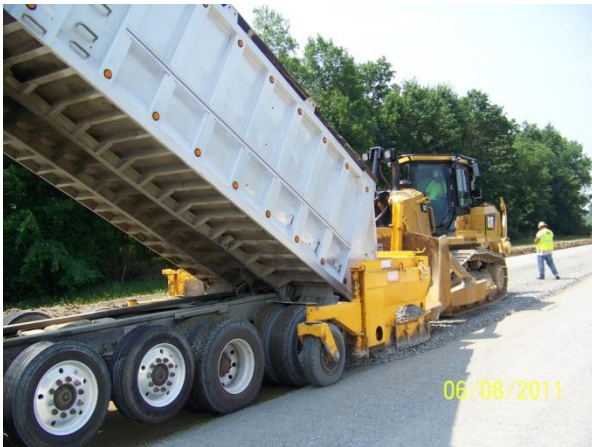
Aggregate Placement on the I-70 lane addition in Clark County
