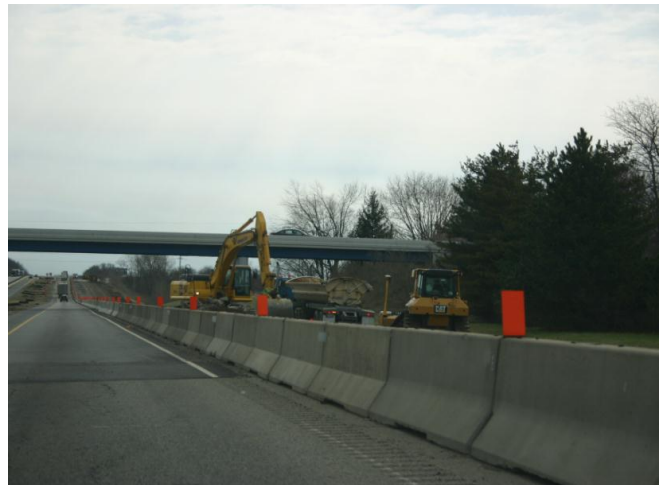
Crews working on the I-70 eastbound lane addition in Clark County
