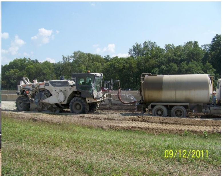
Cement Stabilization on Clark IR70 Project
