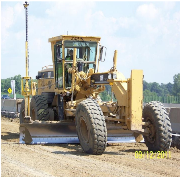
Fine Grading Subgrade on Clark IR70 Project
