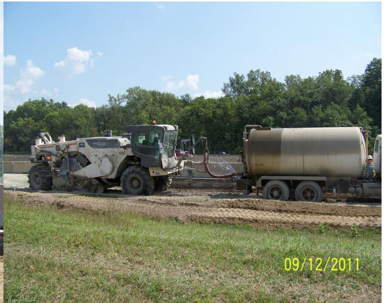
Cement Stabilization On Clark IR70 Project
