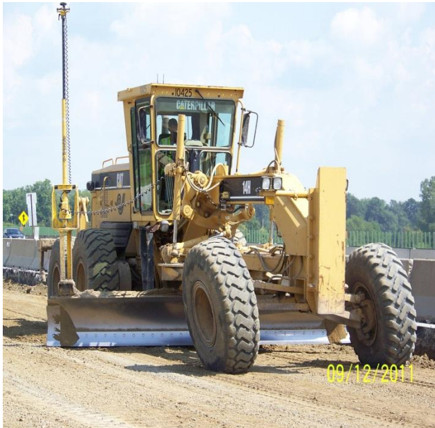
Fine Grading Subgrade On Clark IR70 Project
