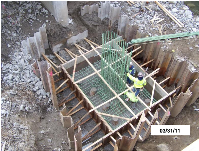
Construction of a pier footer on the Hole's Creek bridge
