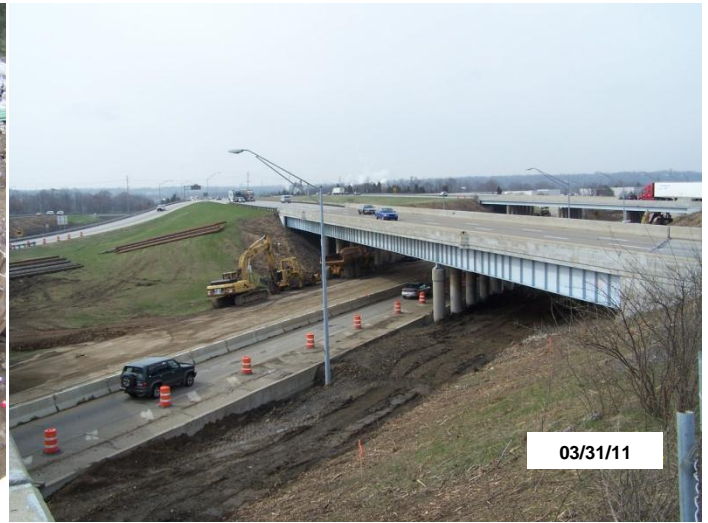
Looking south at I-75 with Central Ave. below
