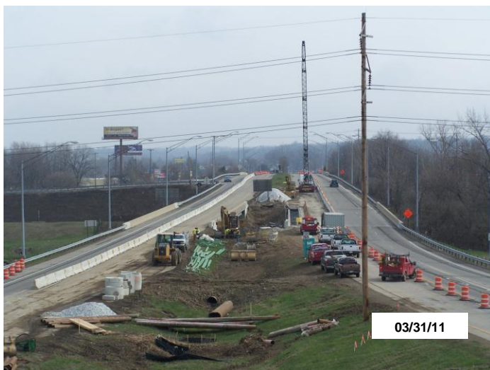
Looking east along Central Ave. & Dixie Dr. from I-75
