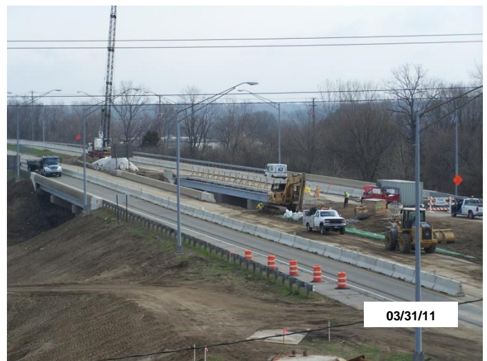
Bridge over Hole's Creek on Central Ave. & Dixie Dr.
