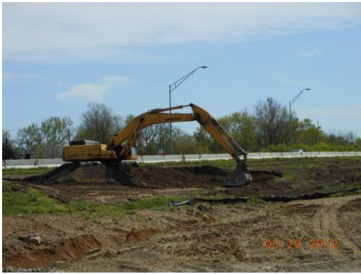
Excavation near where the new northbound I-75 exit ramp will be
