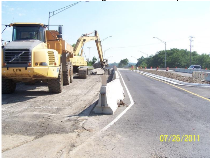
Work on Dixie Dr. near Dryden Rd.
