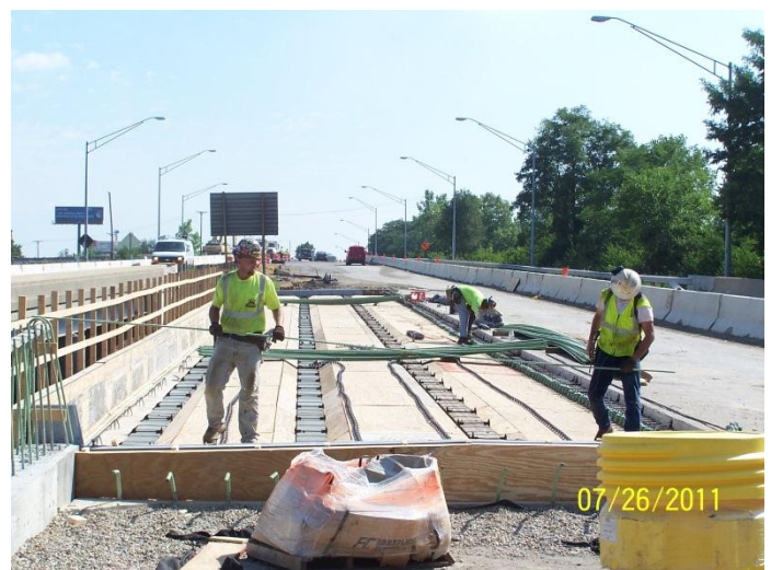
Placing reinforcing steel on the Dixie Ave. bridge over Hole's Creek
