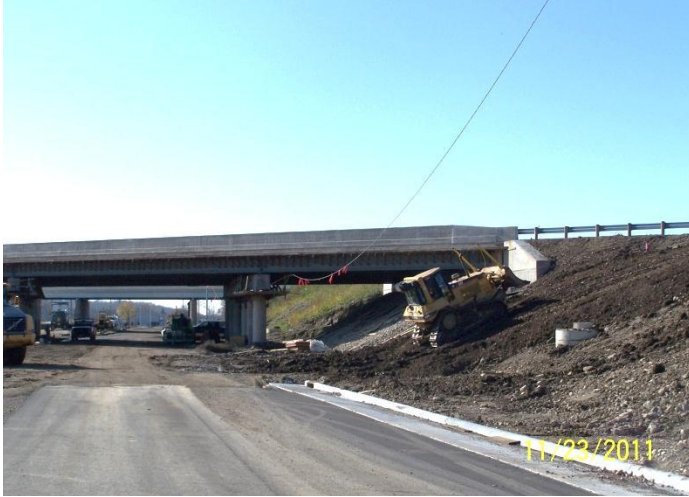
Grading the slope at the I-75 NB bridge over Central Ave.
