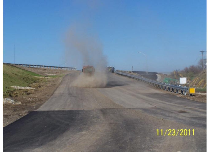
Sweeping off the new ramp from Central Ave. to NB I-75
