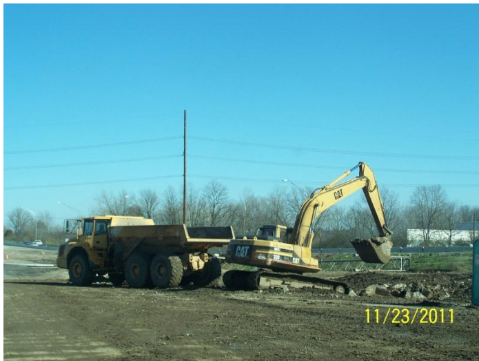
Excavation work between Central Ave. and Dixie Dr. east of I-75
