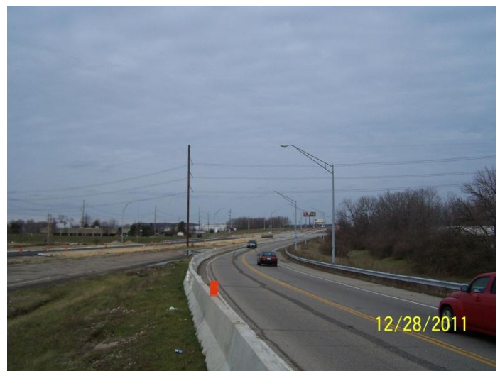
Two way traffic on Dixie Drive, east of I-75 looking east
