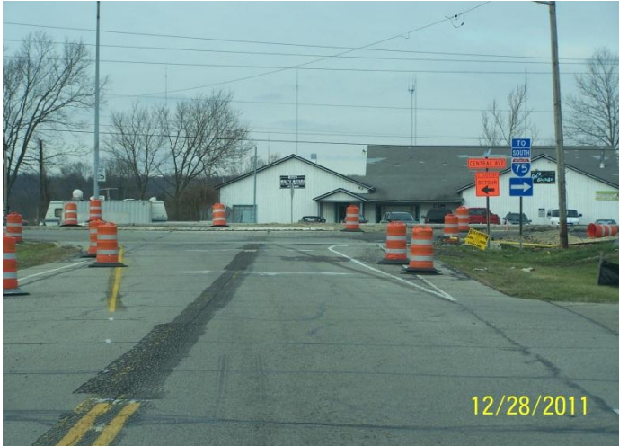
Crossover St. and Central Ave. Going left leads into West Carrollton and right goes to the new ramp to I-75 southbound.
