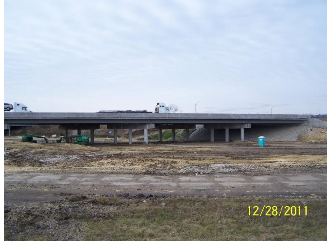
The northbound I-75 bridge over what will become Central Ave. and Dixie Dr.
