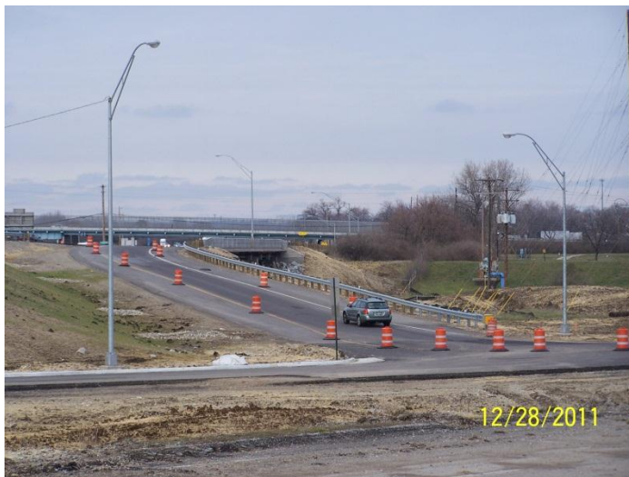
The new ramp from Central Ave. to northbound I-75
