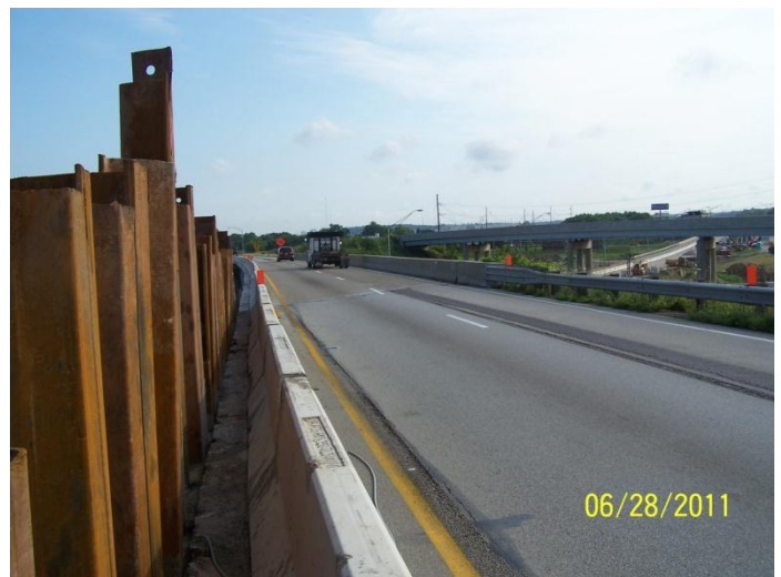
Northbound I-75 at the bridge over Central Ave.
