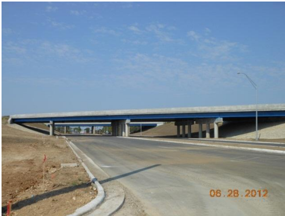
The new southbound I-75 bridge over Dixie Dr.
