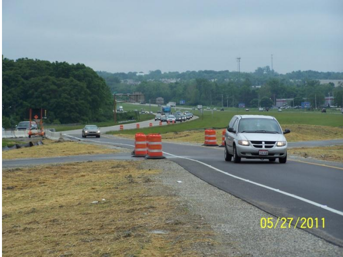
Northbound I-75 traffic using the crossover
