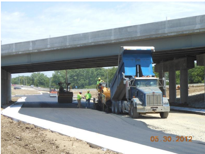
Placing new asphalt on Central Ave. under I-75
