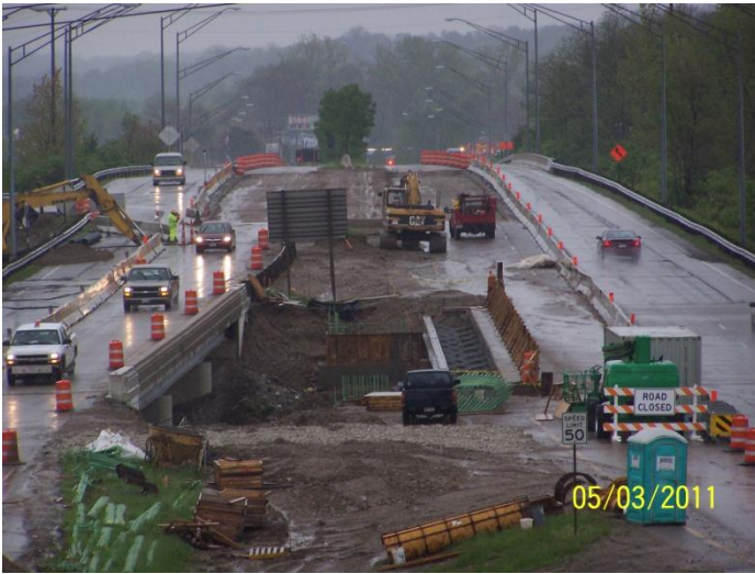
Construction of the Hole's Creek bridge
