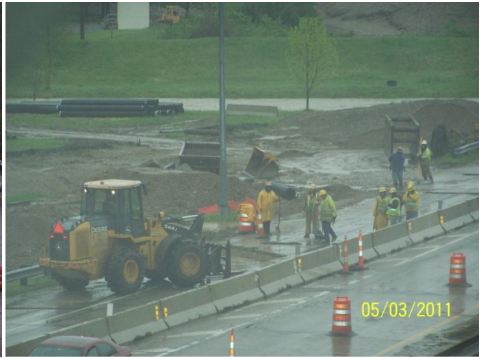
Drainage work on Central Ave.
