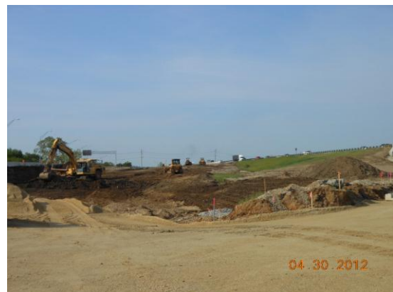
Construction of the new embankment for the northbound I-75 exit ramp
