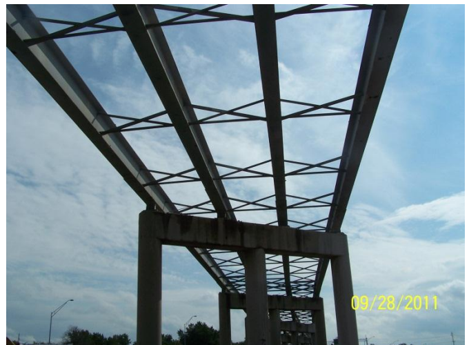
Removal of the old bridge from Dixie Dr. to northbound I-75
