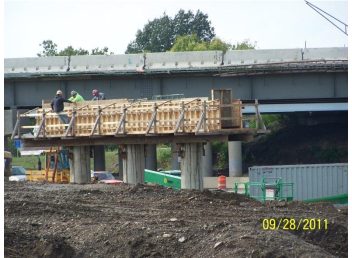
Pouring concrete for the new pier cap for the northbound I-75 bridge over Central Ave.
