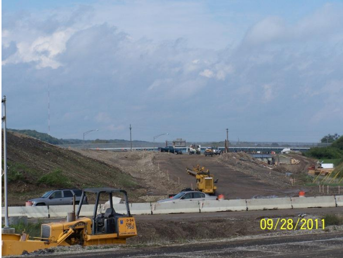
The beginning of the new ramp from Central Ave. to northbound I-75
