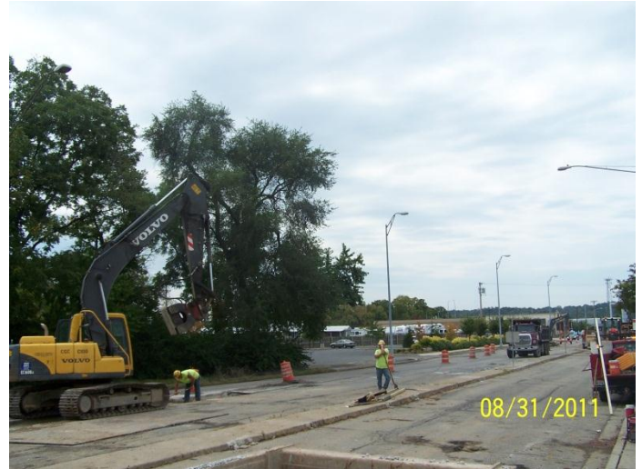
Installing drainage conduit along Dixie Dr. near El Meson
