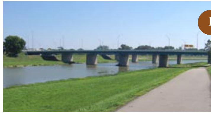
I-75 BRIDGE (SUMMER 2004)
