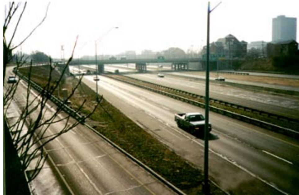
EXISTING OHIO HIGHWAY, I-71 COLUMBUS.
