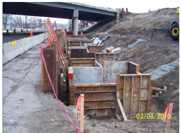
Looking at the third phase of the Keowee Street bridge footer
