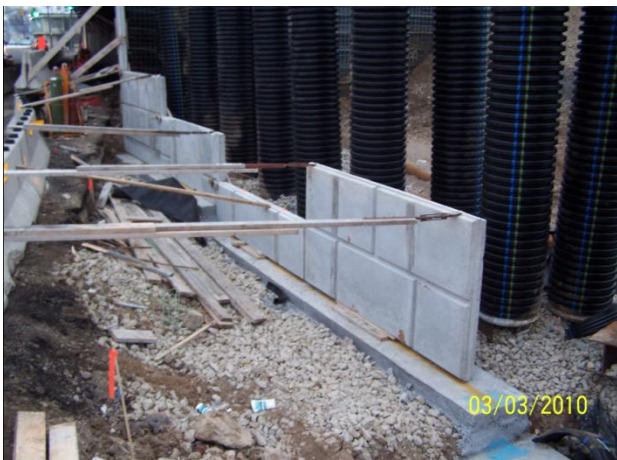
Looking at the MSE Wall 3 along Main Street
