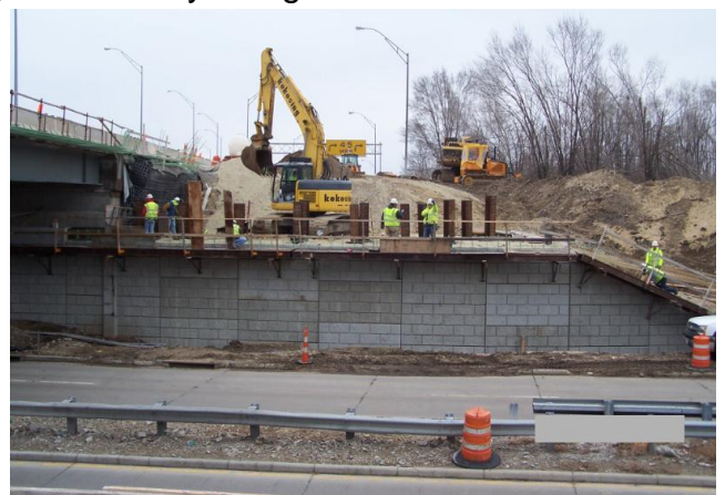
The contractor preparing an MSE Wall for concrete coping
