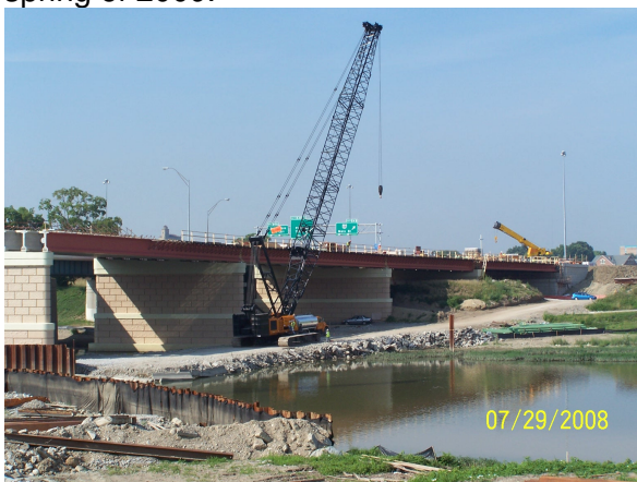
Construction of the bridge over the Great Miami River
