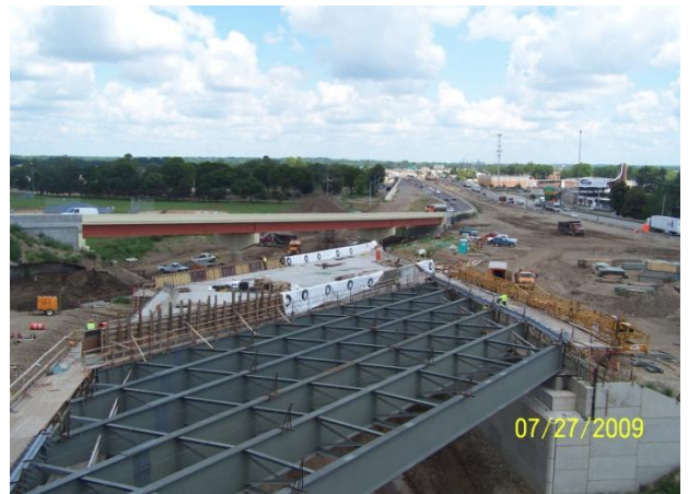
Bridge that will carry traffic from I-75 north and southbound over the exit to State Route 4 north and Webster St.
