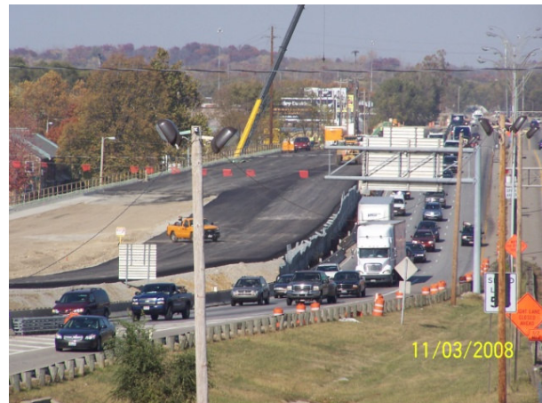
I-75 southbound pavement widening looking north.
