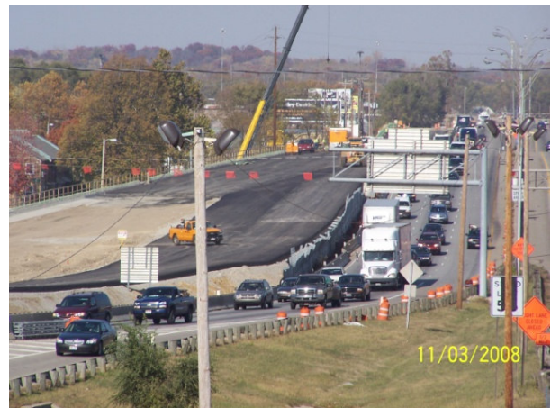
I-75 southbound pavement widening looking north.
