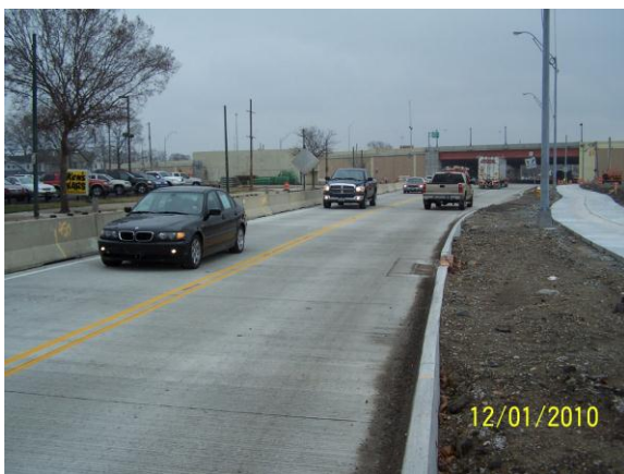
The newly constructed pavement on Main Street
