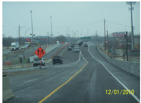
The newly constructed pavement on I-75 NB and the entrance ramp from SR 4 SB to I-75 NB
