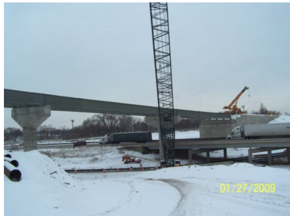
New SR 4 fly-over bridge to I-75 southbound
