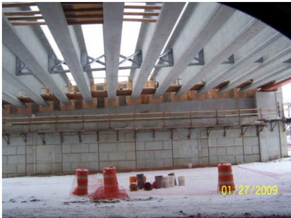
New bridge beams at I-75 southbound over Main Street
