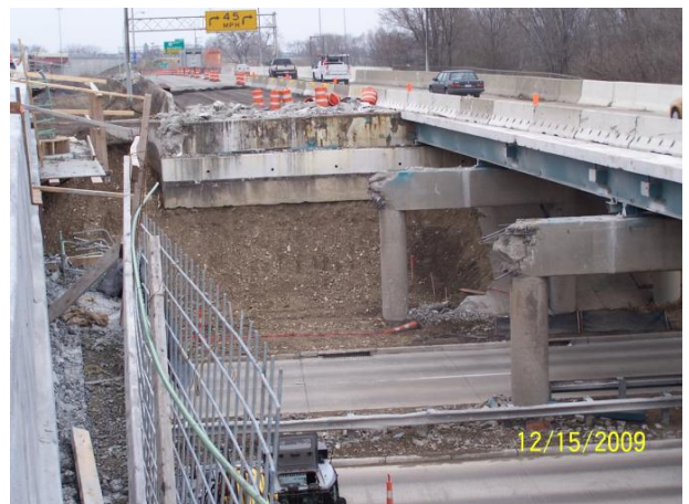
Looking at the new bridge deck over Main St. that is waiting to be poured.
