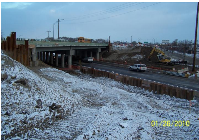
Looking at new construction for a bridge to carry I-75 northbound traffic over Keowee St.
