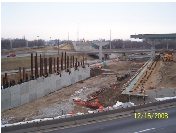
I-75 and SR 4 interchange
