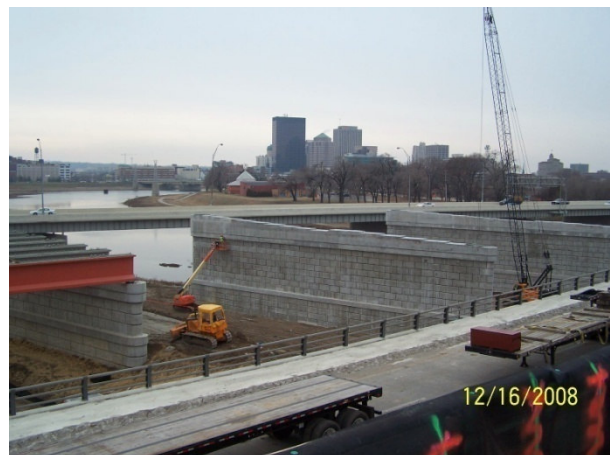
I-75 north and south over the Great Miami River
