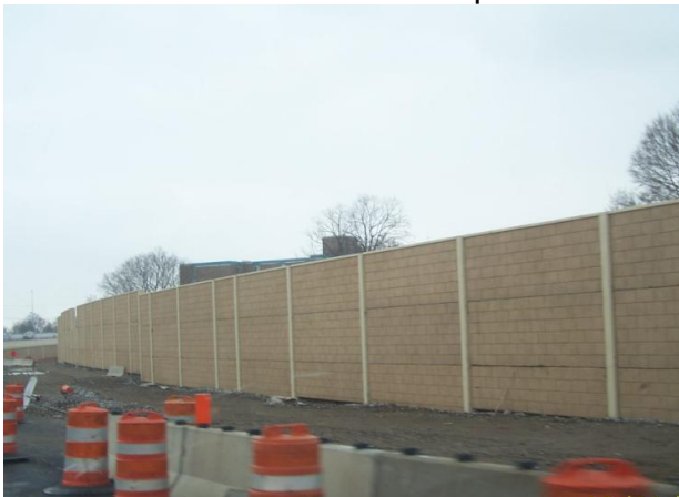
The newly constructed noise wall on the exit ramp from I-75 northbound to Main Street
