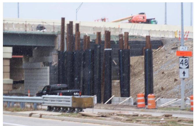
The forward abutment piling at the bridge along Riverside Drive that will carry traffic from I-75 northbound to SR 4 northbound
