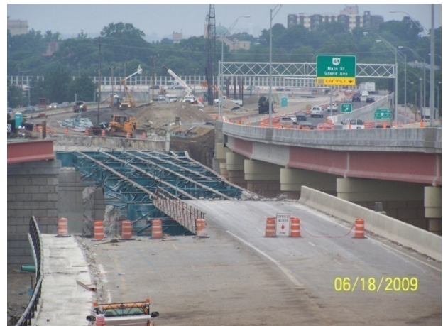
Demolition of the existing I-75 southbound bridge over the Great
