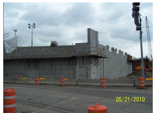
Looking at the MSE wall 3 on Main Street.
