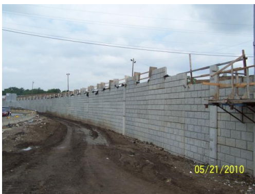
Looking at the MSE wall 2 along the Main Street off ramp.
