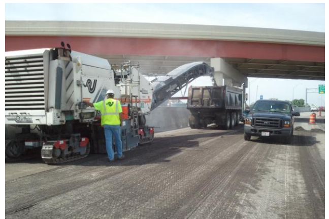
Jurgensen preparing to place new surface course asphalt pavement. .
