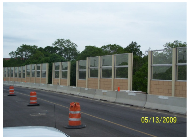
The Main St. on ramp to I-75 southbound noise wall.
