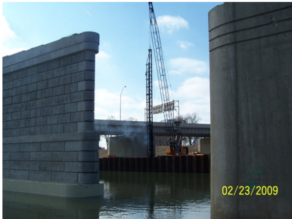
Piling being driven for the I-75 bridge over the Great Miami River
