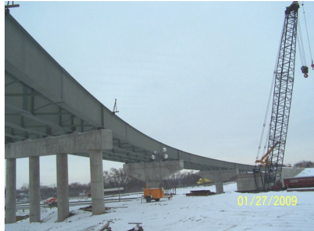
The new flyover bridge from SR 4 southbound to I-75 southbound
