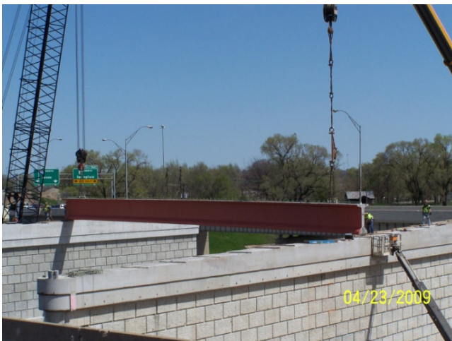
Setting bridge beam for I-75 mainline
