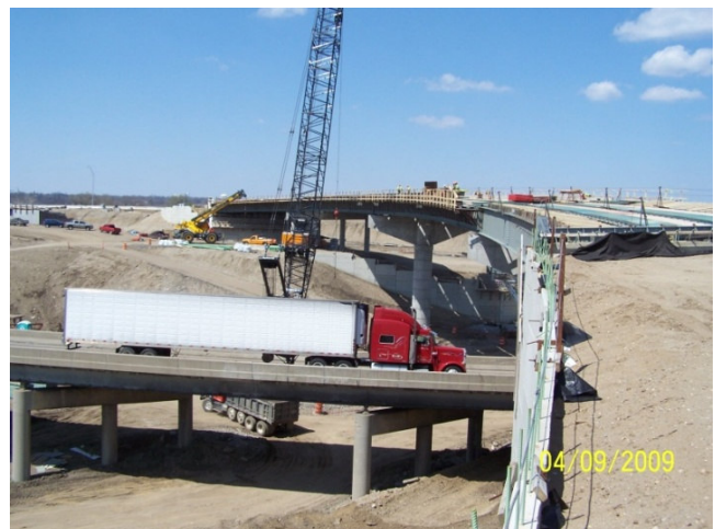
Decking the new flyover bridge over I-75 southbound traffic
