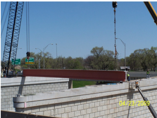
Setting bridge beam for I-75 mainline
