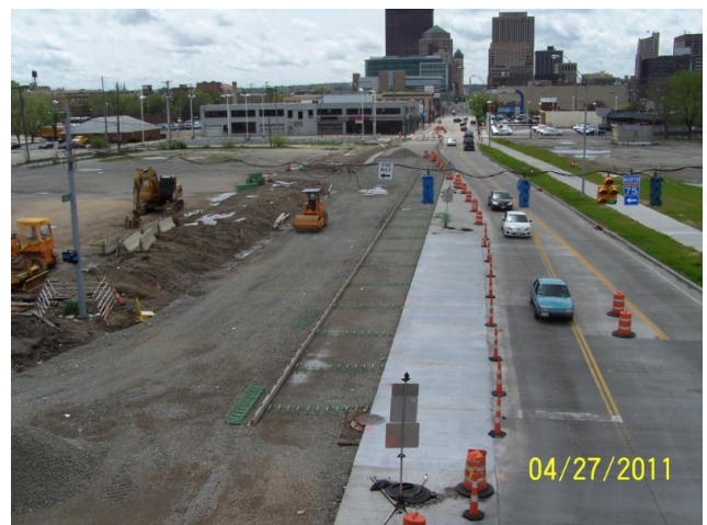
Preparation for Main St. NB lanes concrete pour.
