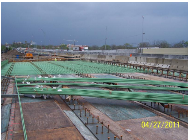
Reinforcing steel installation for the Riverside Dr. bridge deck.
