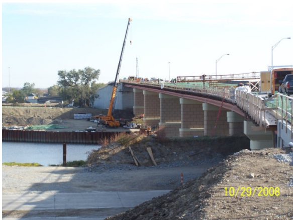
Construction of the Great Miami River Bridge
