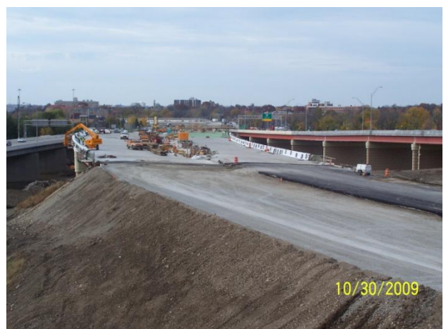
Looking at the bridge over the Great Miami River that will carry both north and southbound I-75 traffic.
