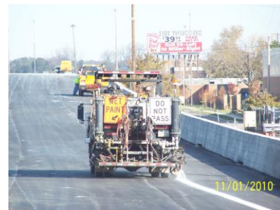
Looking at new striping along I-75 NB
