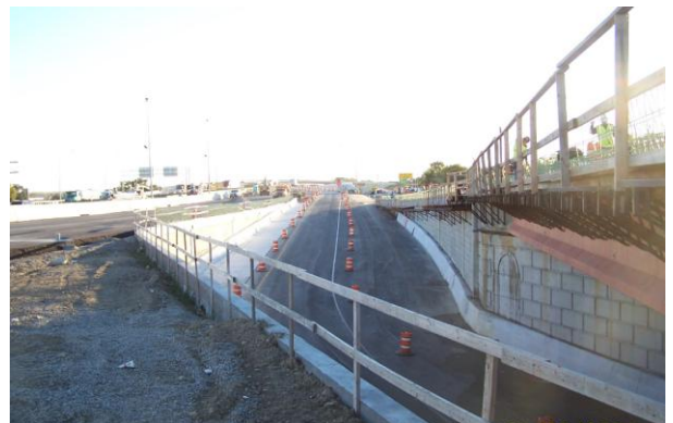
Looking at the new ramp from Main St. to I-75 NB.
